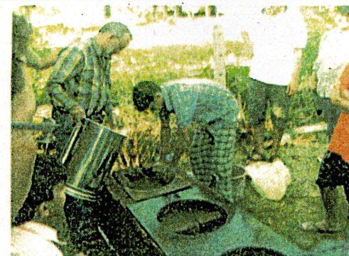
Image 2.1: Making a smokeless fireplace which consumes 70 per cent less fire wood
